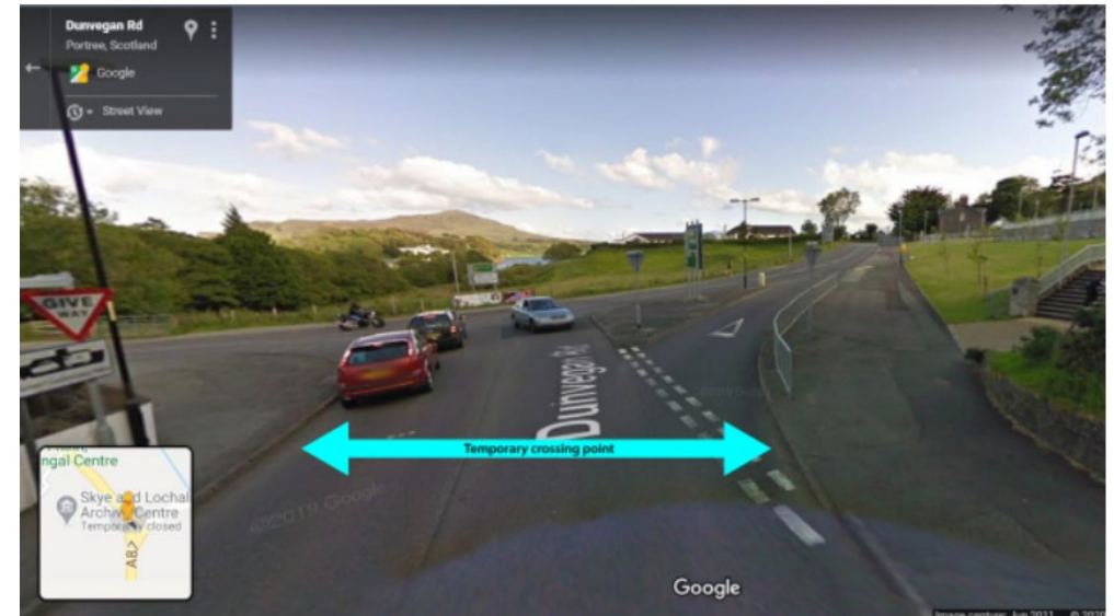
Temporary lights-controlled crossing point on Dunvegan Road
